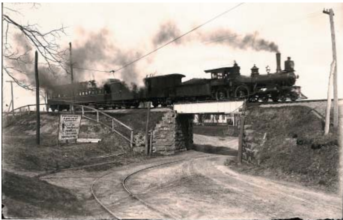
In this photo, dated 1898, a train runs on the old bridge over Lovefield Street. The sign before the bridge reads: Your Money Back if goods are not satisfactory. Clothe Your Boys at Hubbell's Cash Clothier Northampton. (photo courtesy the Easthampton Historical Society)
