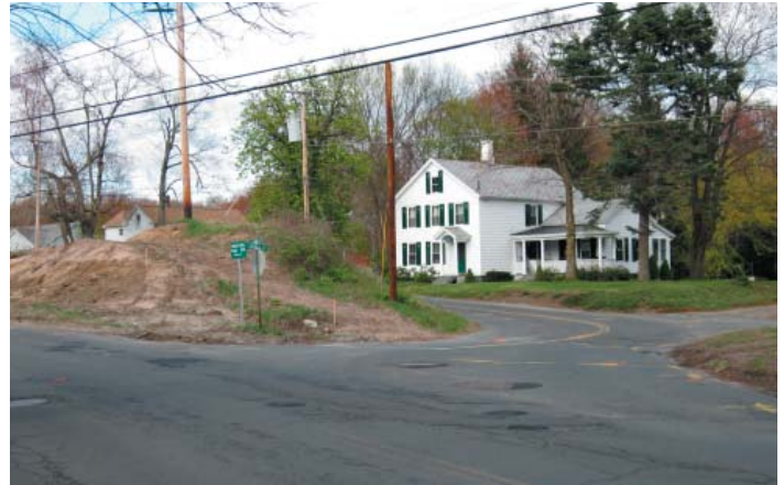
This photo, taken April 2010, shows the remnants of the old bridge abutment. The earth, once built up to support the tracks, will be leveled somewhat to accommodate the new section of the Manhan Rail Trail.
