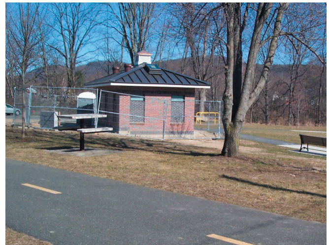
Rest rooms have been built at the Lower Mill Pond Park along the Manhan Rail Trail near Ferry Street. This spring a band shell will be installed overlooking the pond allowing for summertime concerts at the park. The park also includes basketball courts, a childrens play area and an exercise circuit. A grand opening for the park is tentatively planned for June 19th.
